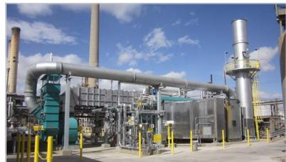
and efficient boiler solution. Nationwide Boiler was the only supplier that could provide a new, in stock 200,000 lb/hr Babcock and Wilcox FM120-124 750 psig design pressure, 750F superheat design temperature package boiler complete with a low NOx burner available for quick delivery.
